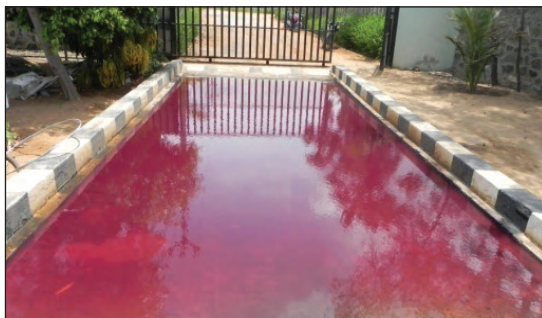
Compound Wall and Vehicle Tyre Wash in L. vannamei hatcheries
