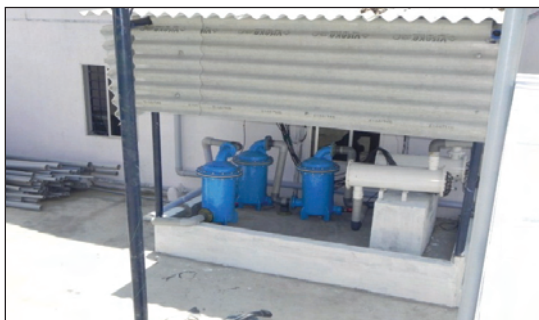
Water treatment and filtration systems in L. vannamei hatcheries
