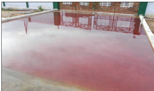
Compound Wall and Vehicle Tyre Wash in L. vannamei hatcheries
