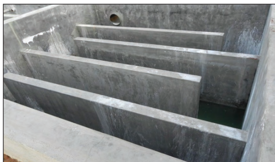
Baffle Walls and Effluent Treatment System in L. vannamei hatcheries
