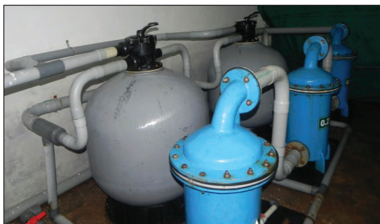
Water treatment and filtration systems in L. vannamei hatcheries
